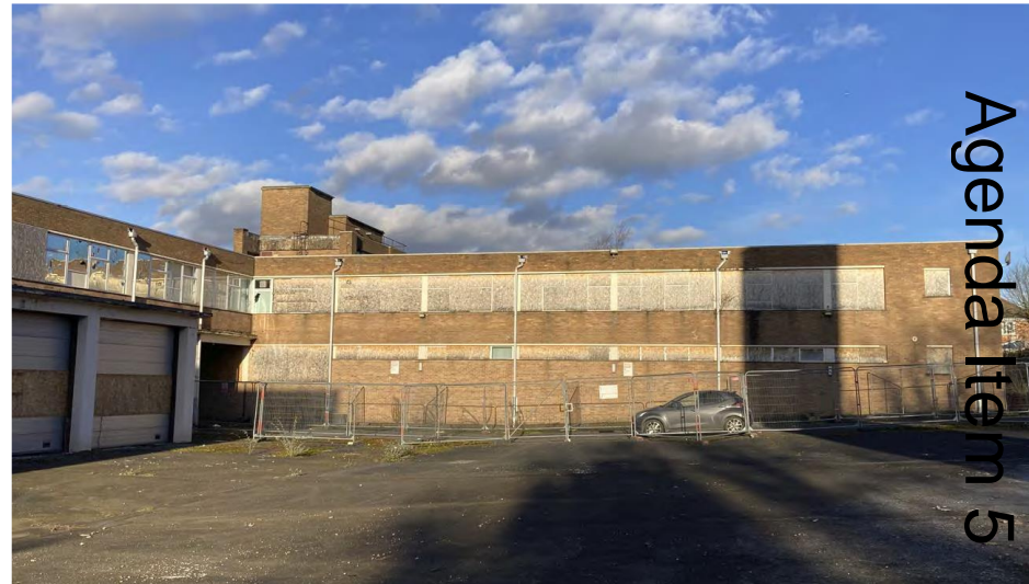
View of rear of Fire Station from courtyard hardstanding area
