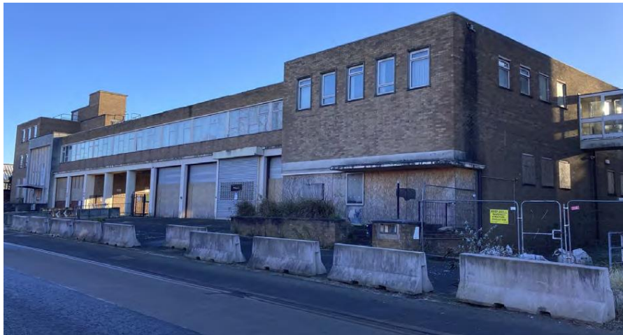
View from Windsor Street of Office Block and Fire Station
