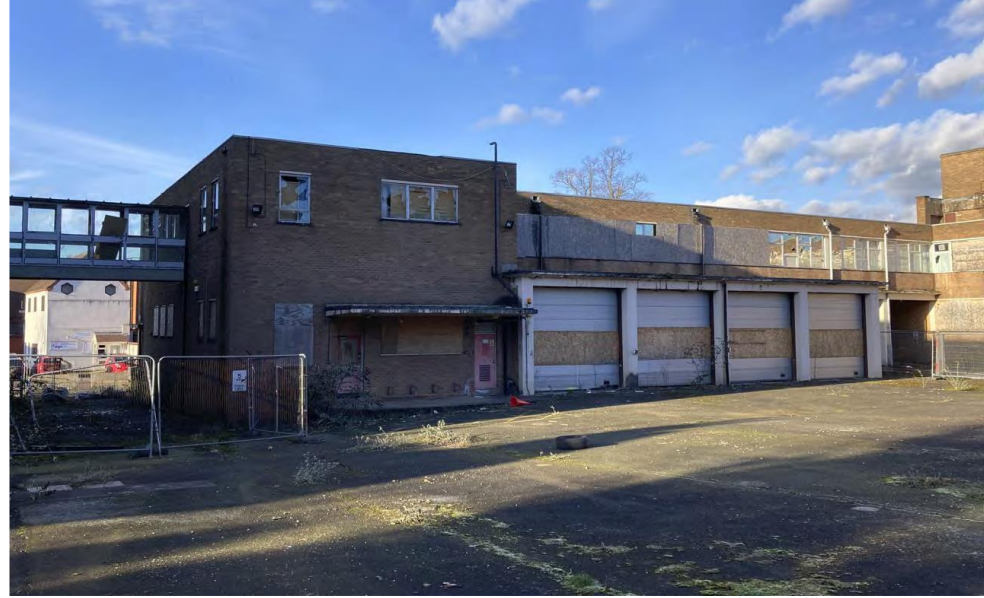
View of Office Block / Library from courtyard hardstanding area
